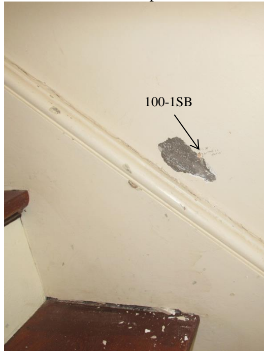
Plaster Wainscot Sample Location
